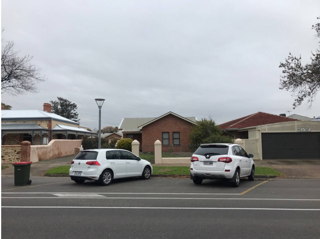
Figure 8: Subject allotment at 151A Childers Street, North Adelaide (centre)
